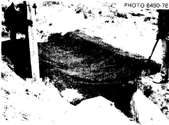
Fig. 12.2. Tamping earth over edge of a side trench of Rug-Covered Trench Shelter at 15 psi.
